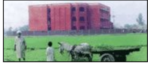
Hoping for education - a TCF building under construction.
