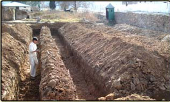
TCF Primary school under construction in Oghi, Mansehra
